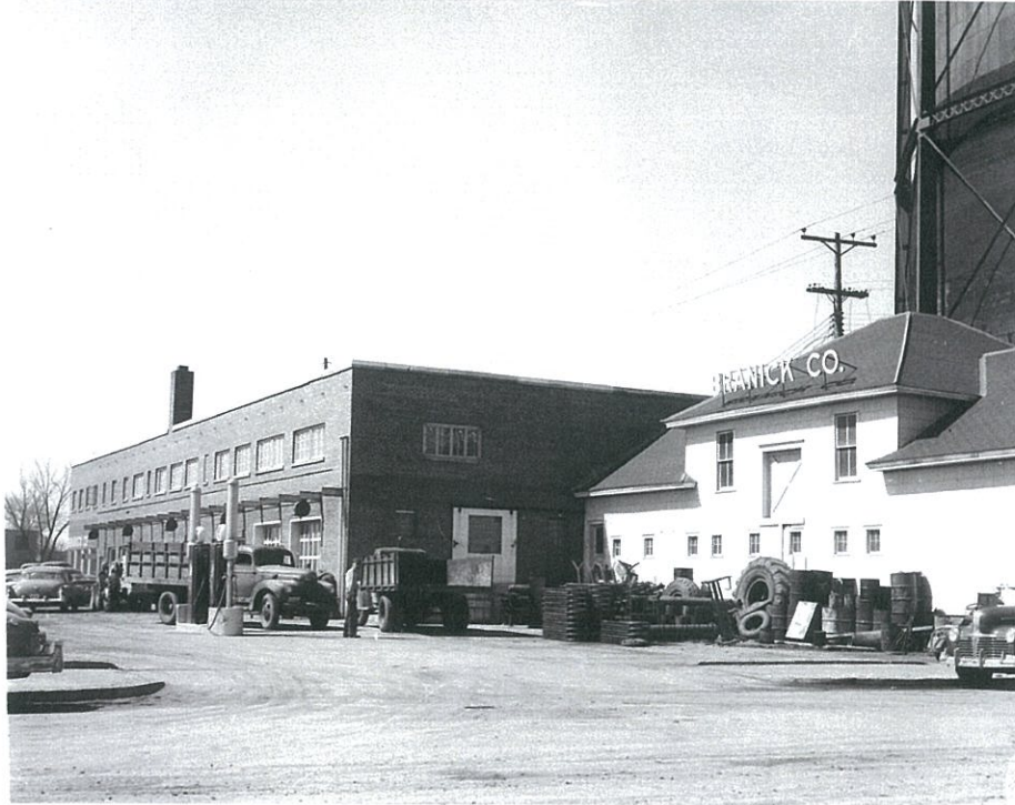
South East Corner (1950 – 1957)
