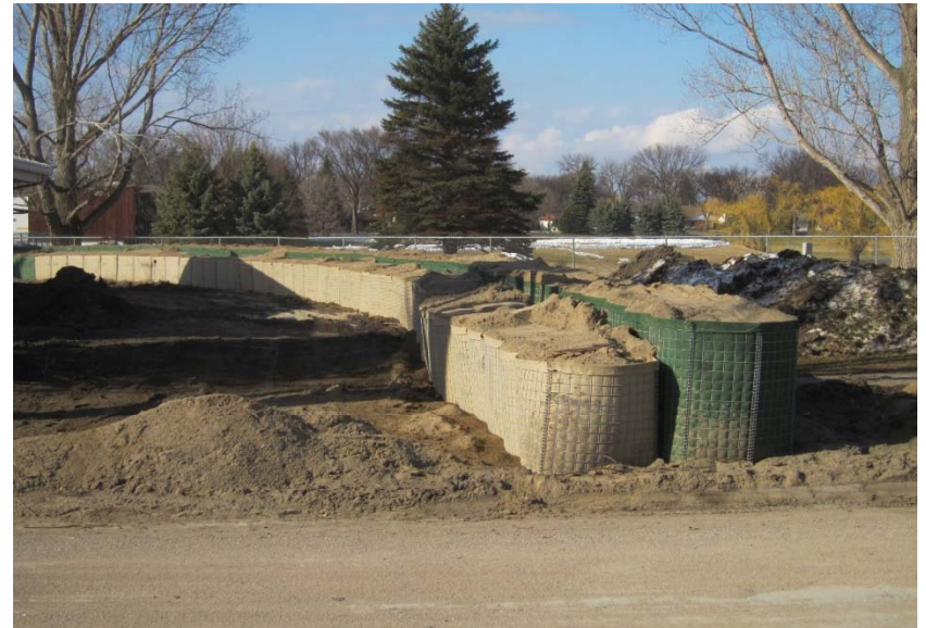
April 6, 2011: A double-barrier of Hesco dikes lines the west side of El Zagal Golf Course at 14th Ave. N in Fargo, ND. Red River stage (at Fargo): 32.5'.
