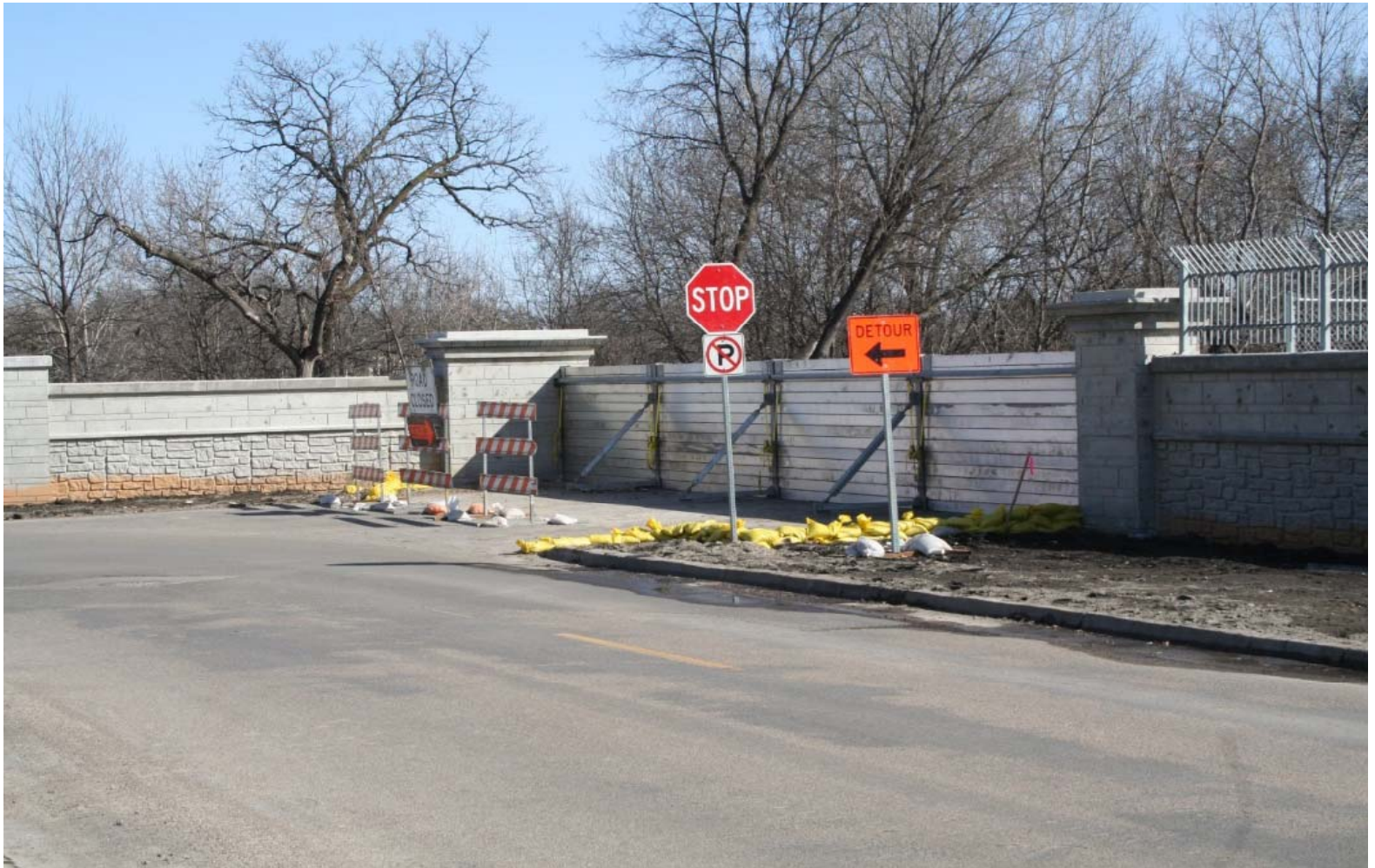
March 21, 2010: Elm Street at 15th Ave. N at flood crest. Flood barricades of the new flood wall (completed 2009) are working effectively. Red River stage (at Fargo): 36.99'.
