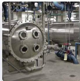
After softening, the water is disinfected with ozone gas and then filtered to remove fine particles, additional hardness, and dissolved minerals like iron. All EPA standards for water clarity were met for 2012. Finally, chloramine is added before distribution to provide disinfection right up to the tap in Fargo homes.
