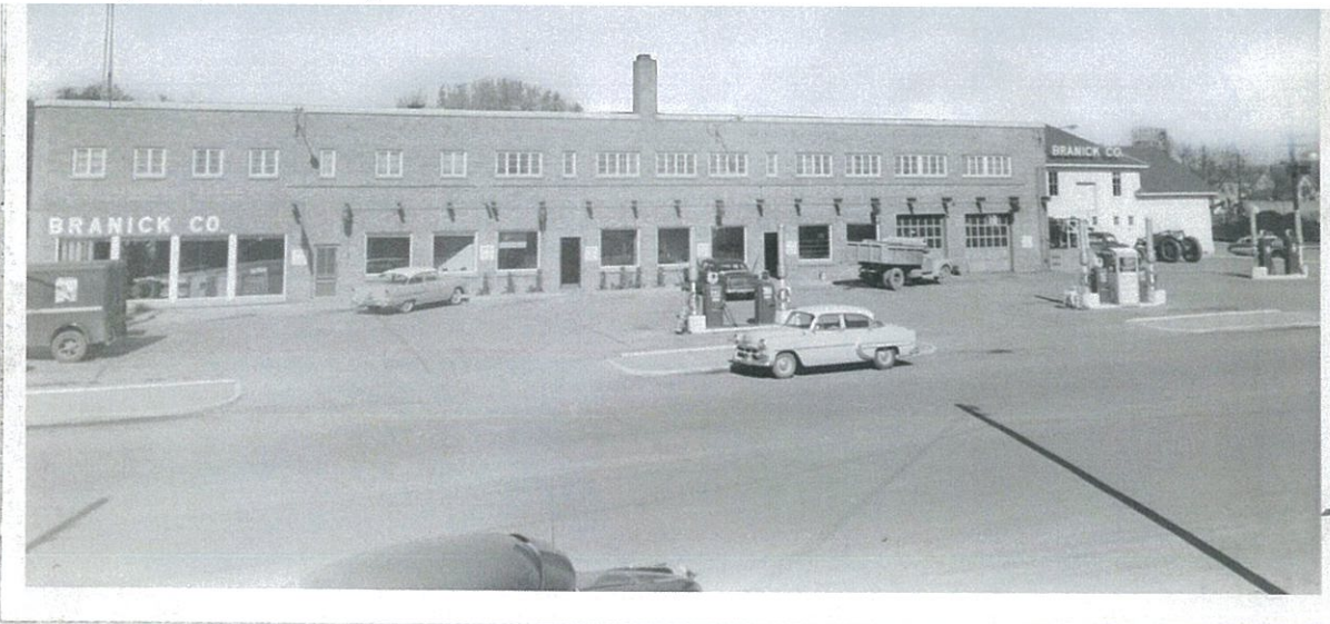
South East Corner (1950 - 1957)
