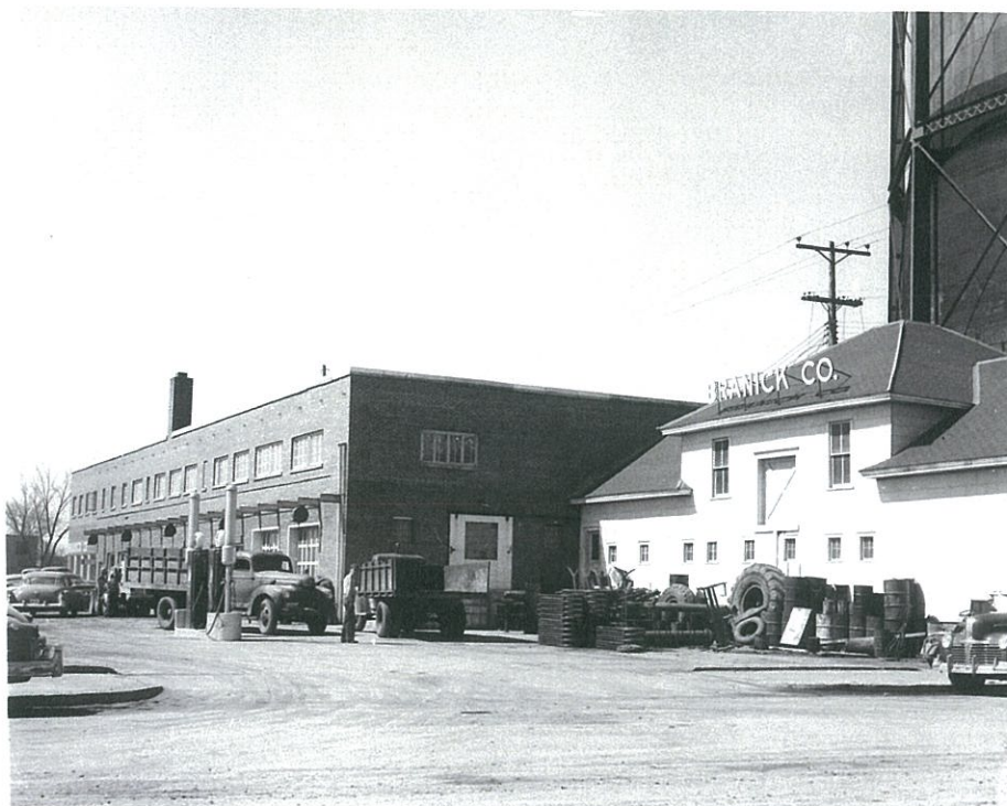
South East Corner (1950 – 1957)
